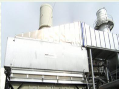
**Energy Savings Potential** - The available heat in a boiler's exhaust gases is dependent upon the hydrogen content of the fuel, the fuel firing rate, the percent of excess oxygen in the flue gases, and the stack gas temperature.
